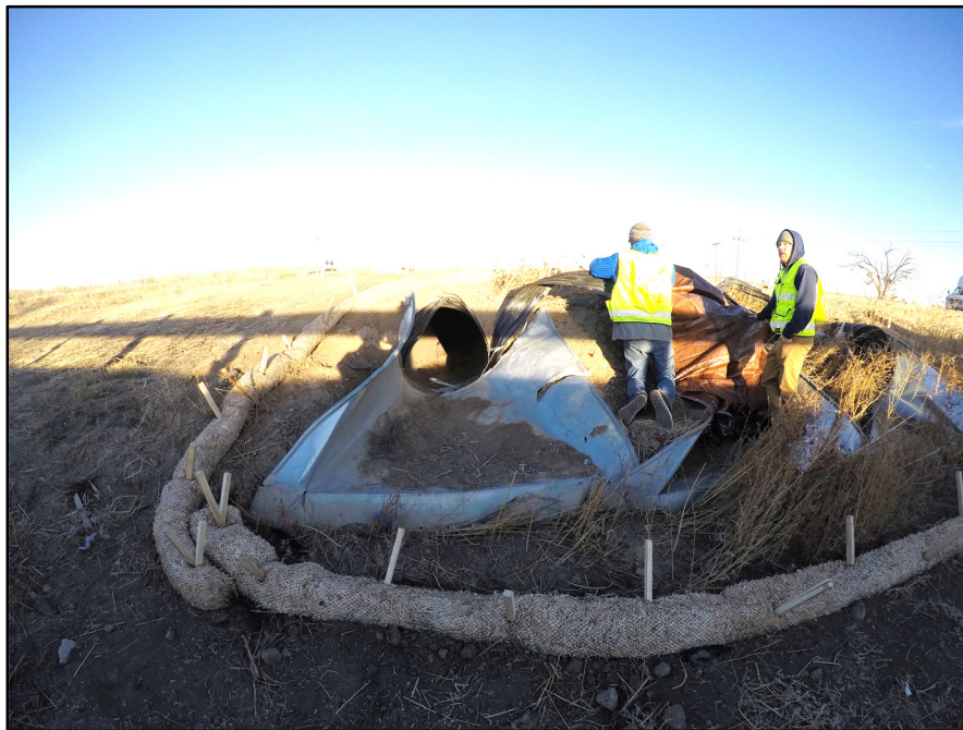
Figure 4412. Manual inspection of I-25 HDPE cross-culverts near Colorado Springs
