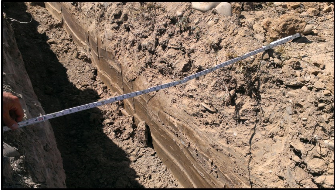
Figure 28. Trench dimensions for HDPE pipe installation
