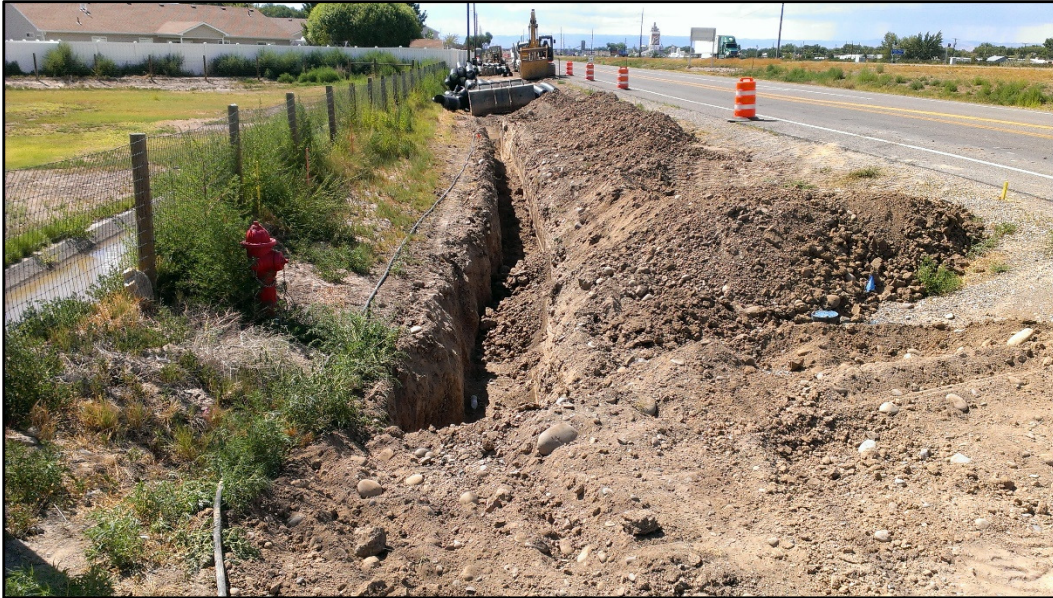
Figure 26. Preparation for the installation of a 3,000-ft HDPE pipeline
