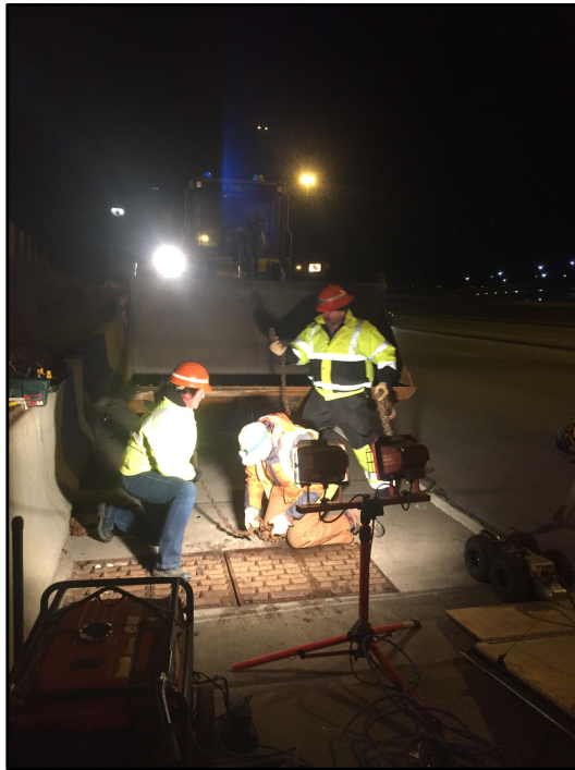
Figure 39. CDOT Maintenance crew providing access to T-Rex HDPE site
