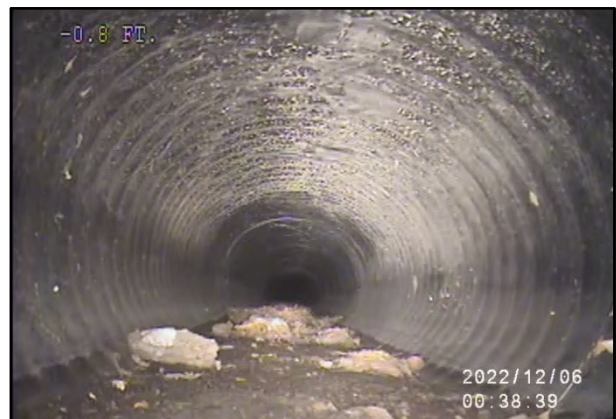
Figure 21. CCTV inspection of an HDPE pipe under CDOT T-Rex project
