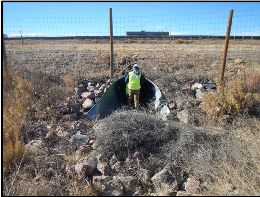
Figure 32. Pipe inspection site near Colorado Springs, CDOT Region 2
