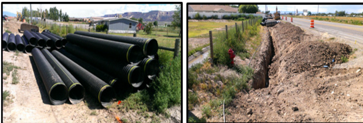
Figures 1 and 2. Typical HDPE installation project in Colorado
