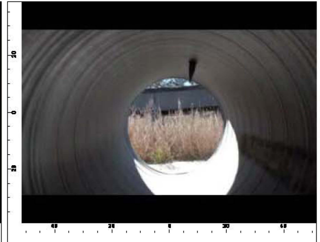
View of erosion control stake through crown of structure.
