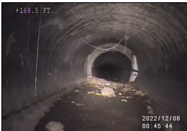
Figure 10. CCTV inspection of an HDPE pipe under CDOT T-Rex project
