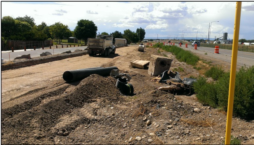
Figure 27.8 Preparation for the installation of a 3,000-ft HDPE pipeline
