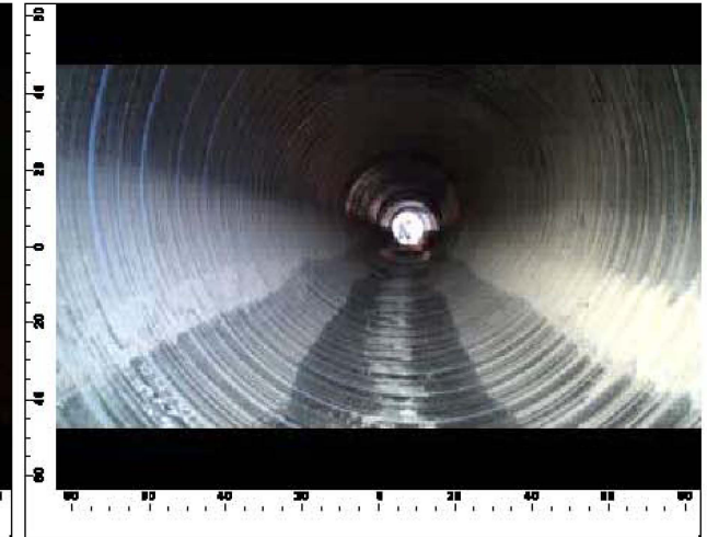
View from outlet end, pipe slight racked near outlet end not caught by laser.
