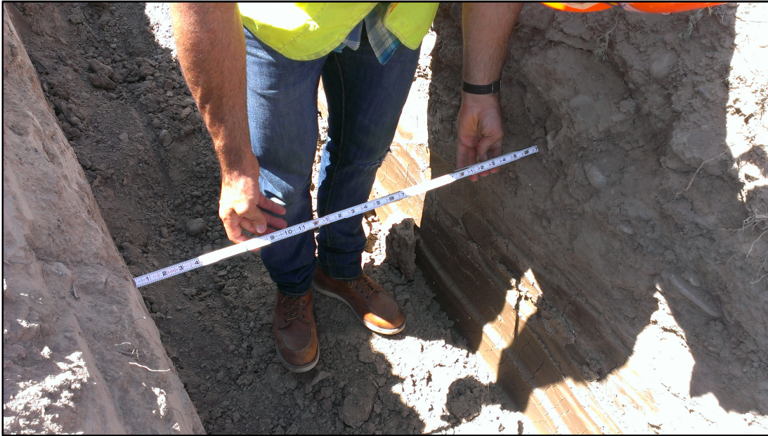
Figure 30. Trench dimensions for HDPE pipe installation
