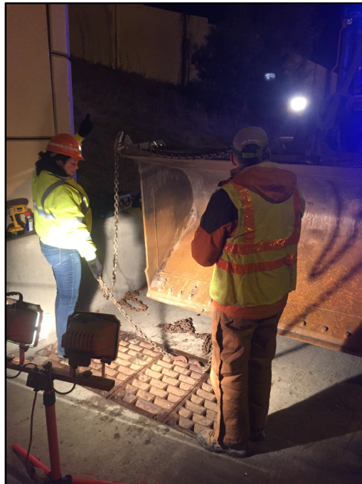
Figure 40. CDOT Maintenance crew providing access to T-Rex HDPE site
