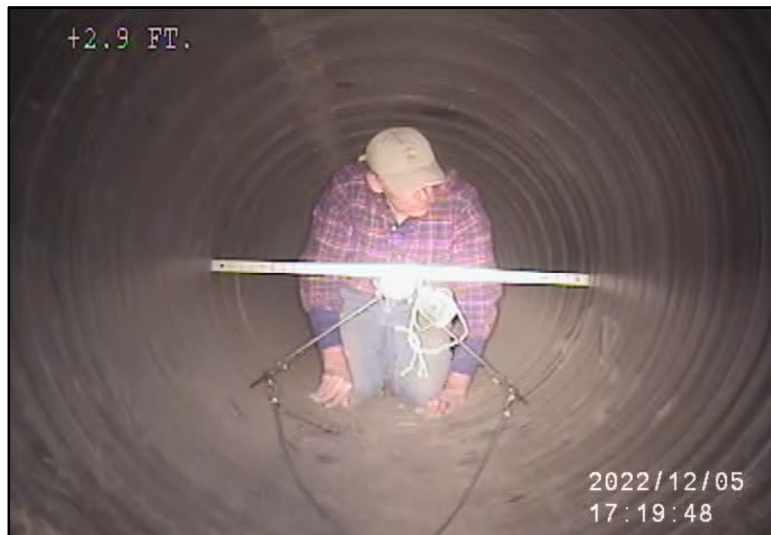
Figure 14. Setting up for laser-ring equipment inside an HDPE pipe under I-25
