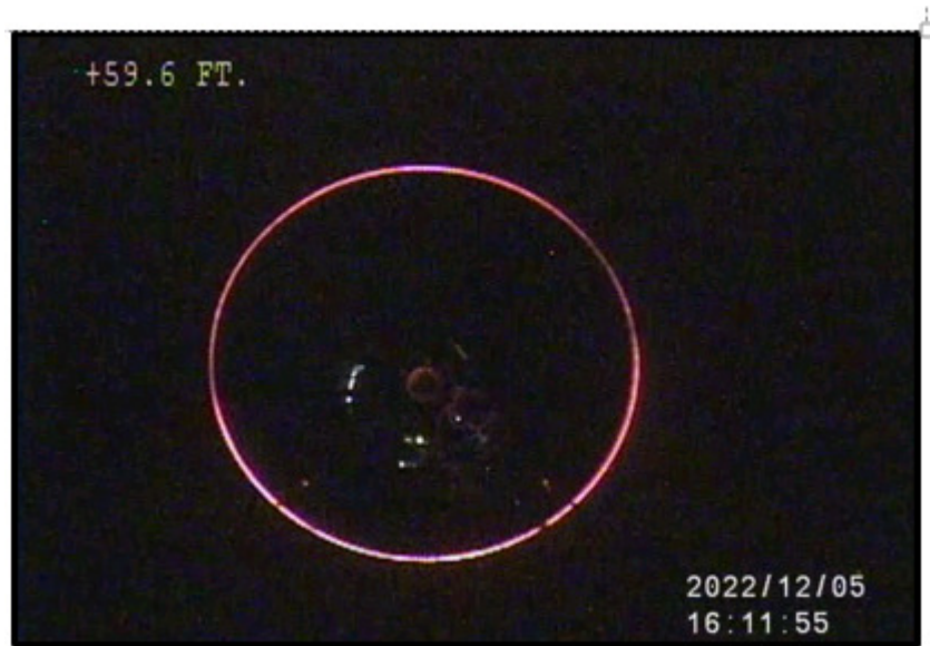
Figure 25. Laser ring reflected on the pipe surface under Interstate 25 at Fountain Creek
