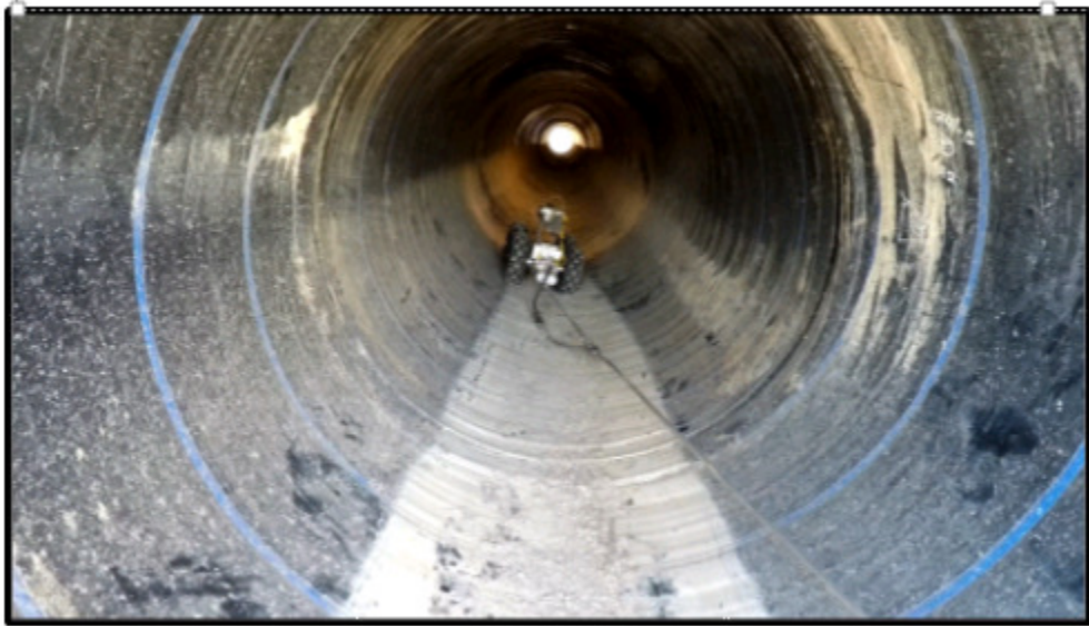
Figure 24. Mobilizing the robotic trolley during the inspection process
