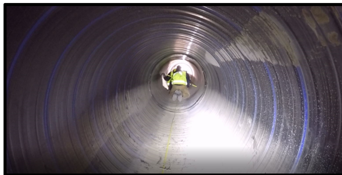
Figure 4. Manual inspection of HDPE pipes
