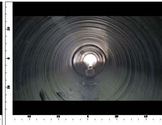
View of pipe towards outlet end of the structure. Pipe appears to be round and uniform.
