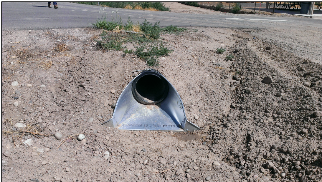
Figure 31. HDPE pipe installation
