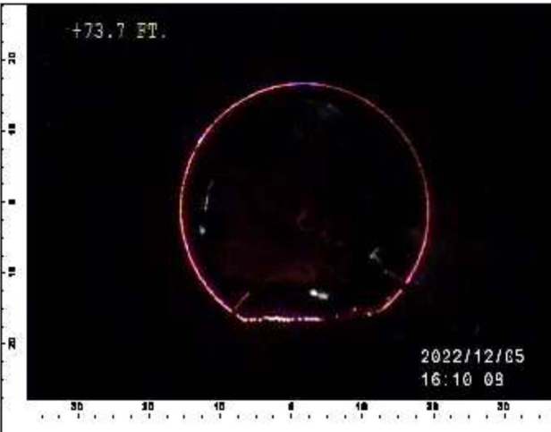
Debris in invert causing spike in vertical data.
