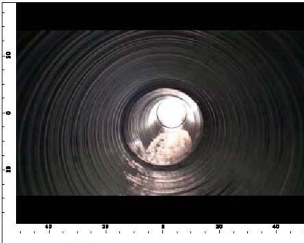
View of second joint.
