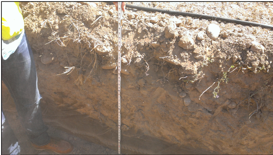
Figure 29. Trench dimensions for HDPE pipe installation
